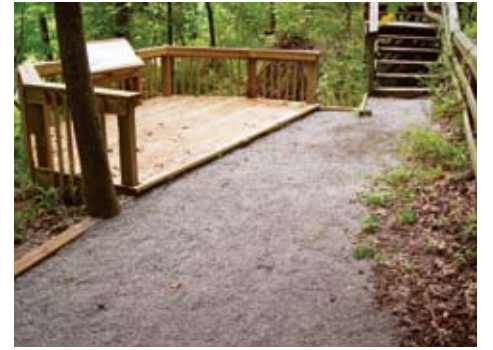
RETAINING WALLS AND GRAVEL
